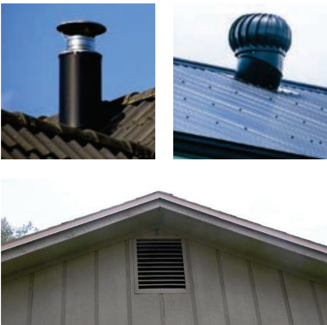
Different types of roof openings that can be used for stack ventilation
